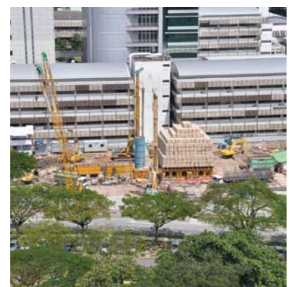
Drilling and pile testing May 2009
